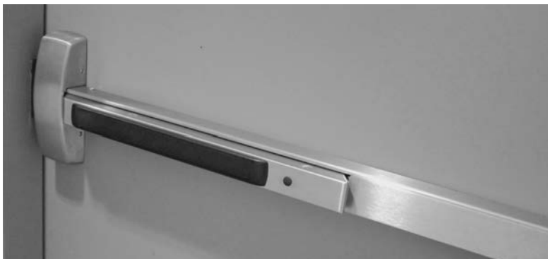
FIGURE 2.5. Panic Bars on Doors. People fleeing a fire would die if they encountered exit doors that opened inward, because they would keep trying to push them outward, and when that failed, they would push harder. The proper design, now required by law in many places, is to change the design of doors so that they open when pushed. Here is one example: an excellent design strategy for dealing with real behavior by the use of the proper affordances coupled with a graceful signifier, the black bar, which indicates where to push. (Photograph by author at the Ford Design Center, Northwestern University.)
